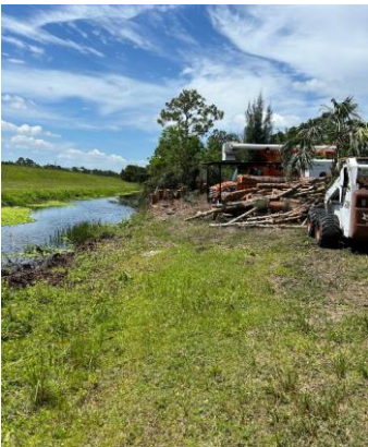
Figure 11. Canal 14 Vegetation Removal
