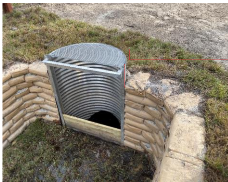
Figure 3. Section 7 Riser/ Culvert Structure
